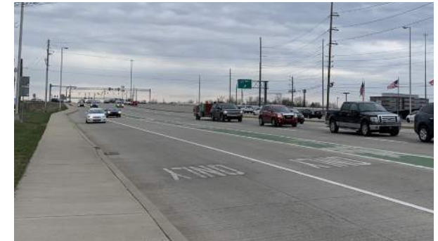
Facing I-465 Intersection (facing south)
