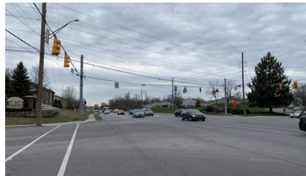
91st Street Intersection (facing south)
