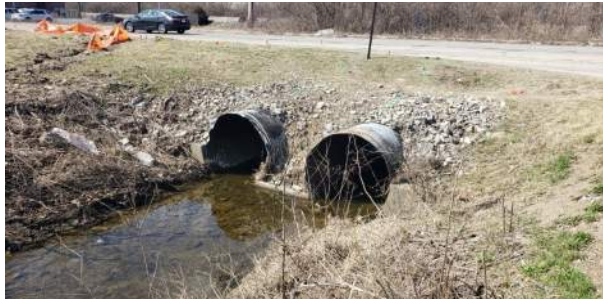
Culvert condition near Castleton Square Mall
