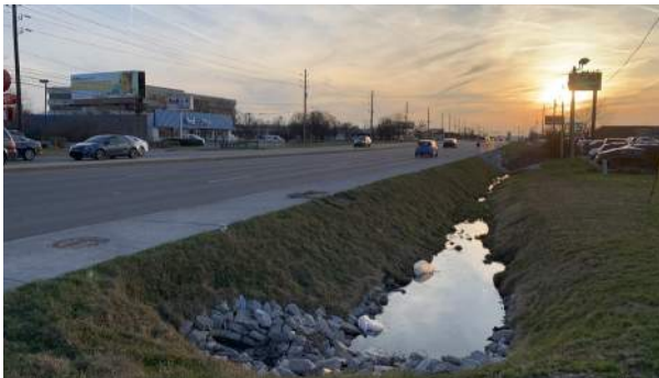
Open drainage on 82nd Street (west)
