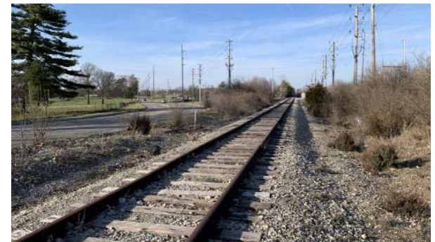
Rail at 86th Street (facing north)
