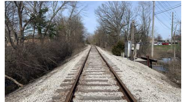
Rail at 75th Street (facing north)
